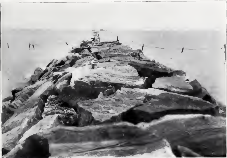
Courtesy War Department. From original photographs in U. S. Engineer's Office CLEVELAND BREAKWATER Showing Final Construction Rough Rubble Work
